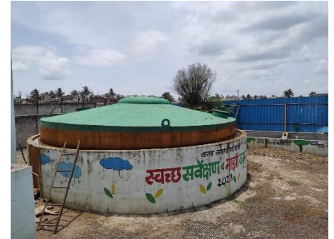
Bio-methanation plant of 5 MT capacity generating 20-22 unit of electricity per day
